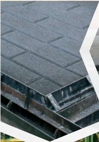
8 Final surface treatment
