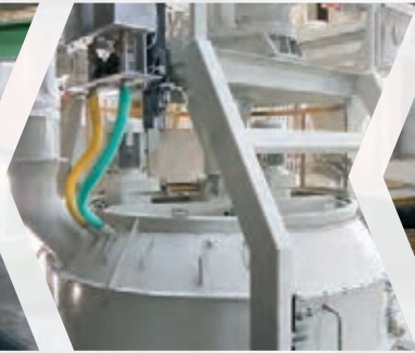
6 Bearing layer concrete mixing
