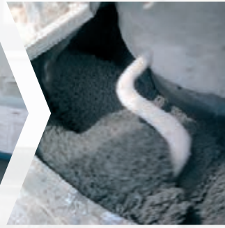
3 Absorbing layer concrete mixing
