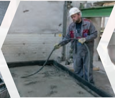
7 Concrete placing and compaction
